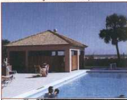
Beach front building before Hurricane Opal.
