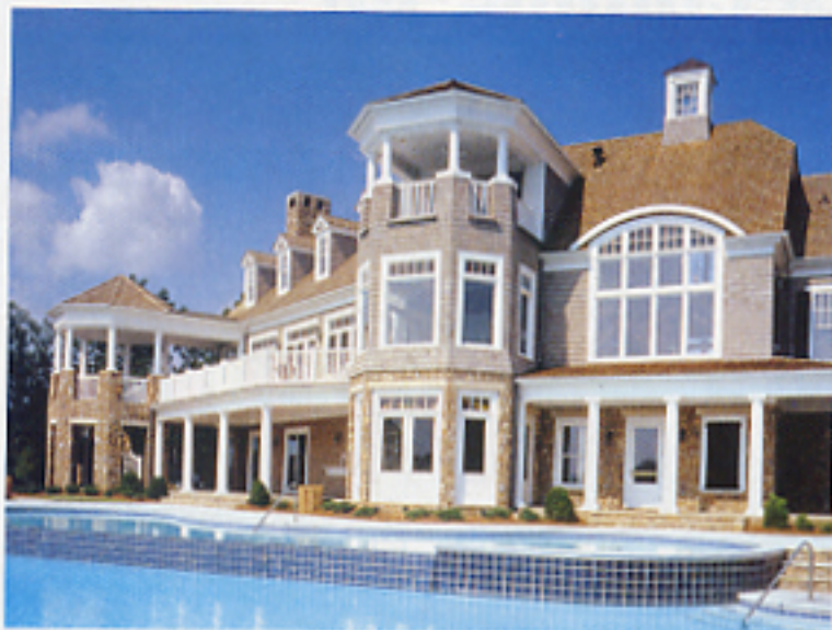
An 8,000 square foot club house and pool is featured at Harbour Point in Atlanta. The roofing is premium Classic pine shingles. (Photos courtesy of LifePine Products LLC.)
